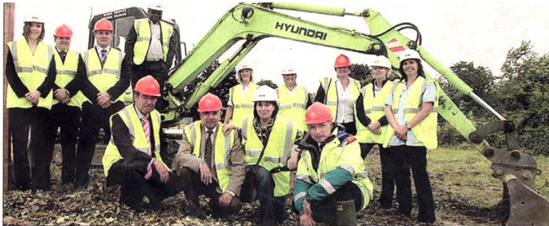
BUILDING WORK: Primary care trust officials, doctors and nursing staff at the site of the soon to be built surgery.
