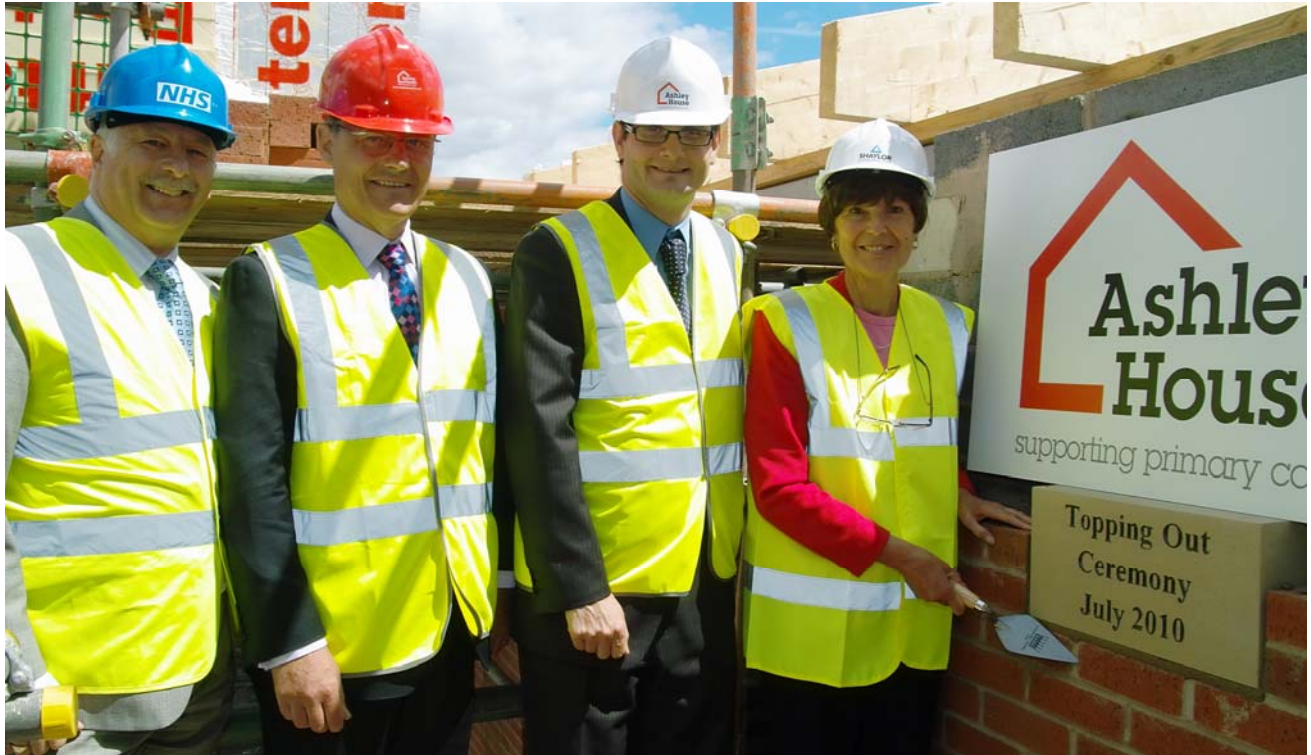
Shown laying the ceremonial foundation stone from left to right; Julian Rainsford, Director of Estates and Facilities, NHS Walsall, David Hartshorne, Chief Operating Officer, Ashley House plc, Dr Geoff Archenhold, Chairman for NHS Walsall and Carol Southall, NHS Walsall Patient
